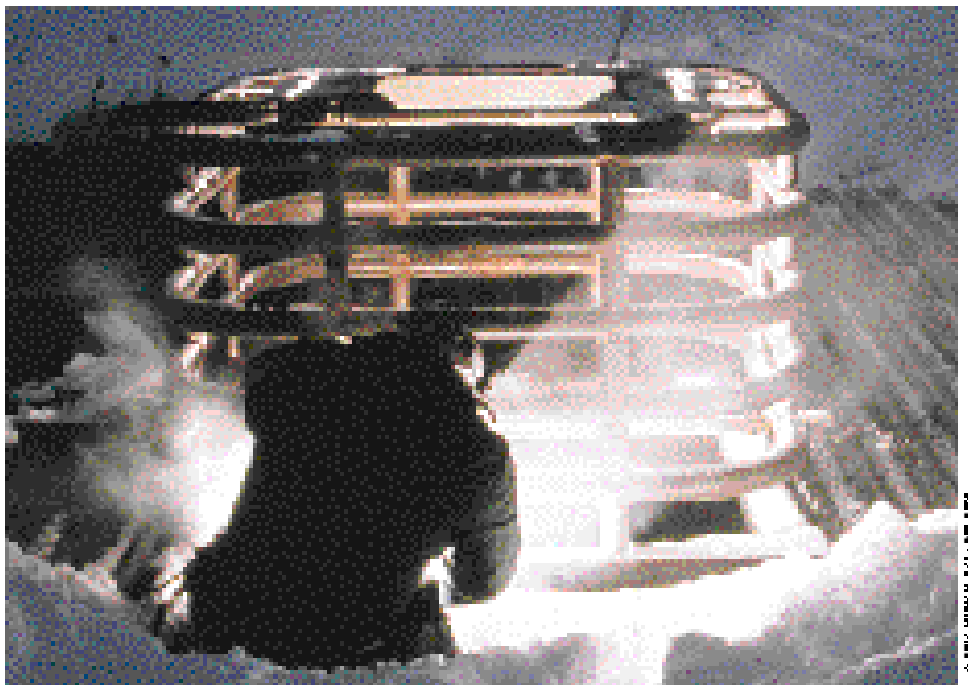
As part of the Great Lakes Bats and Mines Initiative, a new gate is installed at the Pewabic Mine in Michigan, reopening it for use by bats.
